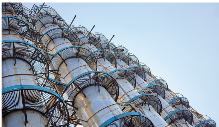
Left: Methanol distillation refinery
